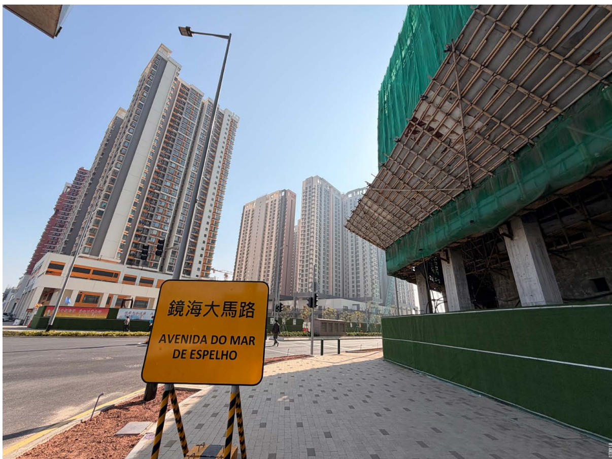
➤ Major roads in Zone A were opened as residents started to move in
